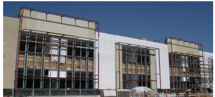
CHS Math & Science Building
