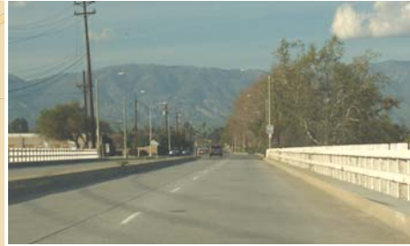
La Cadena / Santa Ana River Bridge
