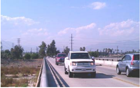
Mt.Vernon Bridge over the Santa Ana River (near the Board Room)
