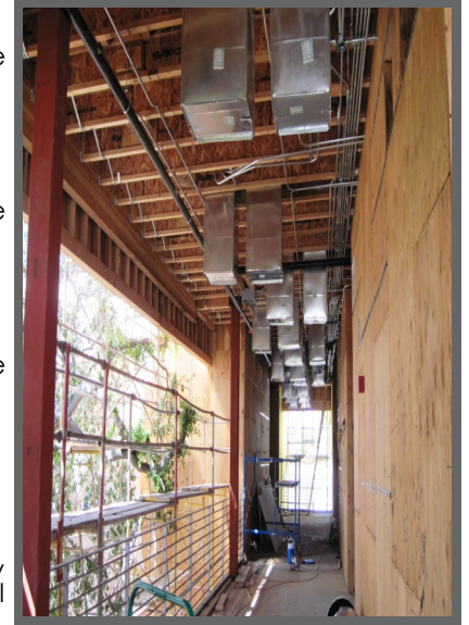
CHS Math & Science Building
