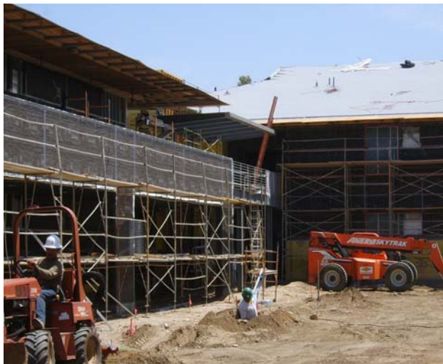
BLOOMINGTON HS MATH & SCIENCE BLDG TOTAL BUDGET: $15.1 MILLION CONSTRUCTION: 53% COMPLETE (+1%)
