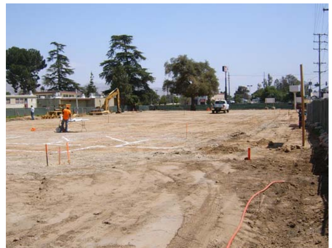
COLTON HS MATH & SCIENCE BLDG TOTAL BUDGET: $18.6 MILLION CONSTRUCTION: 9% COMPLETE (+1%)
